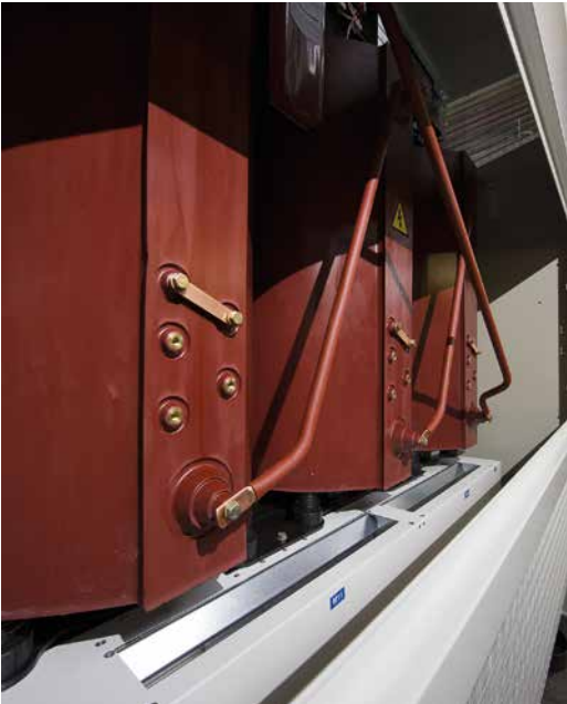
Force-ventilated transformer in IP31 enclosure
